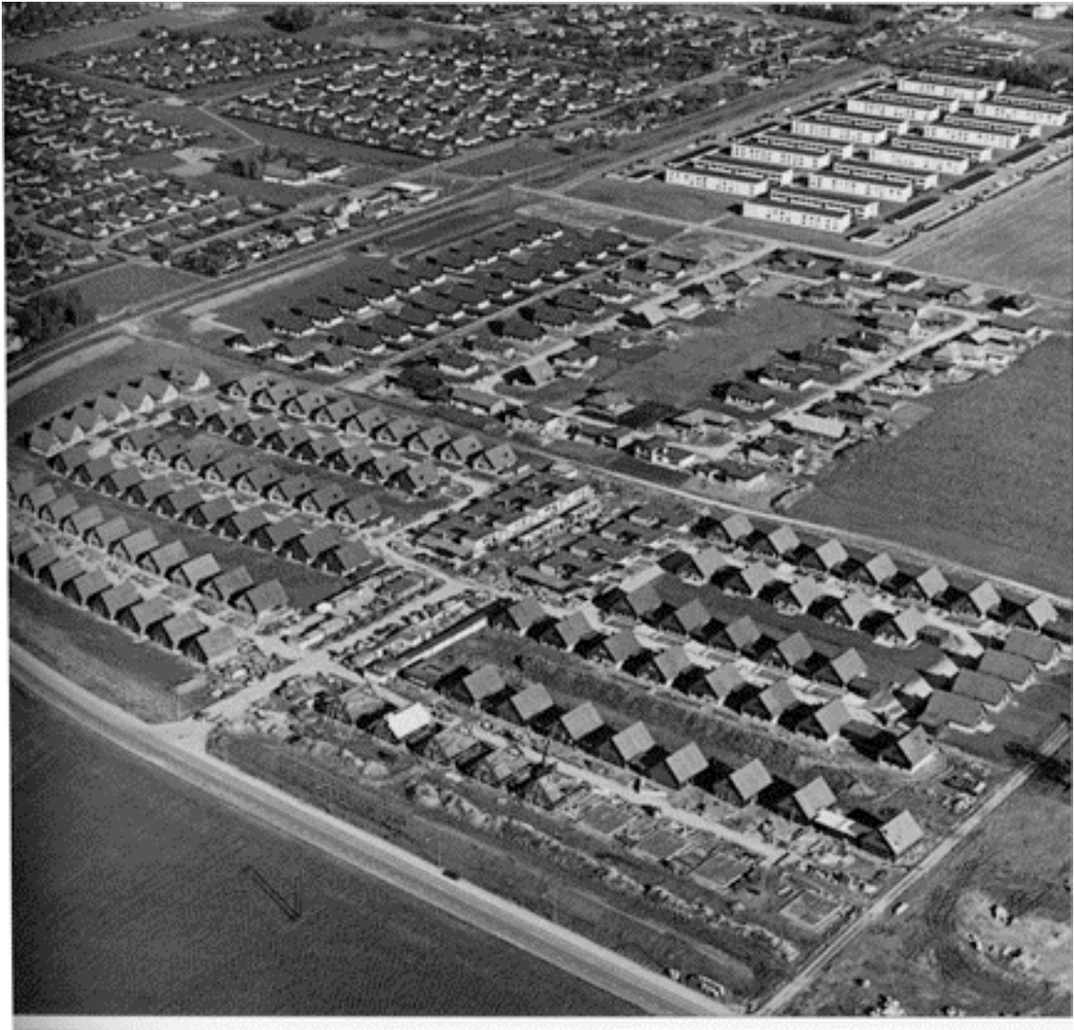
Figure 12.4: The suburb of Staffanstorp, near Lund in southern Sweden, came in the early 1970s to stand as a symbol of the anonymous, housing area with large-scale planning and total adaptation to the car.
