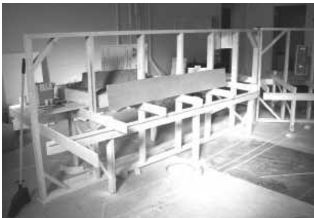
The benchwork for the permanent section of the Upper Mississippi Transportation Corporation began last August.
